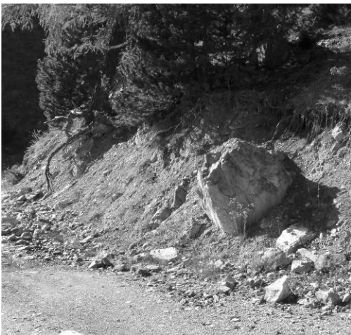
Figure 12 Typical road cut with loose rocks including boulders
