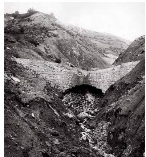
Figure 8 Check dam in the Faucon torrent amidst degraded landscape, pictured from 1901(OMIV-EOST 2009)
