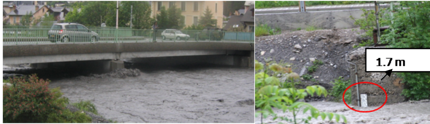
Figure 5. 20. Photograph showing the condition of Abattoir Bridge during the 2008 event (Source :Newspaper 30.05.08, Barcelonnette)
