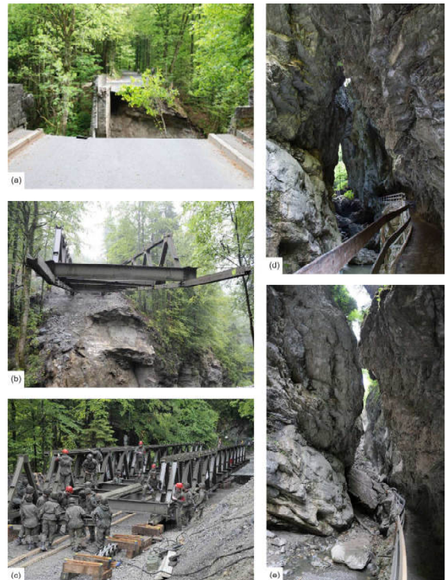
Fig. 2. Impact of the destructive rockfall: (a) the destroyed bridge (photo: Stefan Hoch, source: www.bmlv.gv.at ); (b and c) reconstruction of the bridge by the Federal Armed Forces of Austria (photos: Sigi Schwärzler, source: www.bmlv.gv.at ); (d) view into the gorge in 2010 before the rockfall occurred (photo: Bernhard Mäser) and (e) two days after the rockfall event on 12 May 2011 (photo: Friedrich Böhringer).
